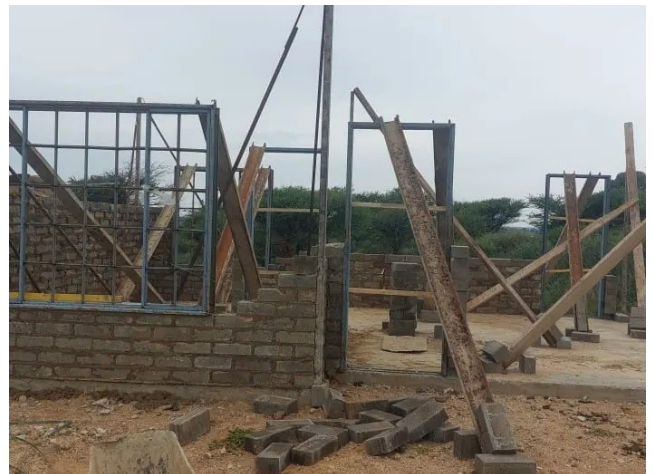
WALLING AND ROOF-FRAME CONSTRUCTION
