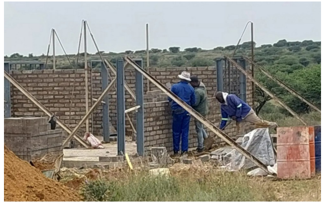
BUILDING WORKS AND STRUCTURAL PROGRESS
