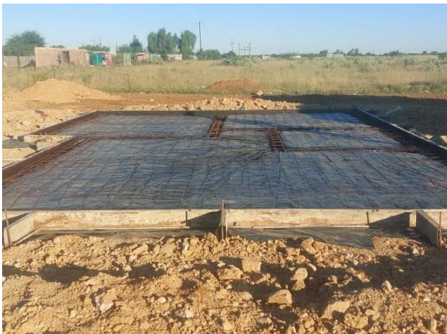
REINFORCED FOUNDATION AND SLAB PREPARATION
