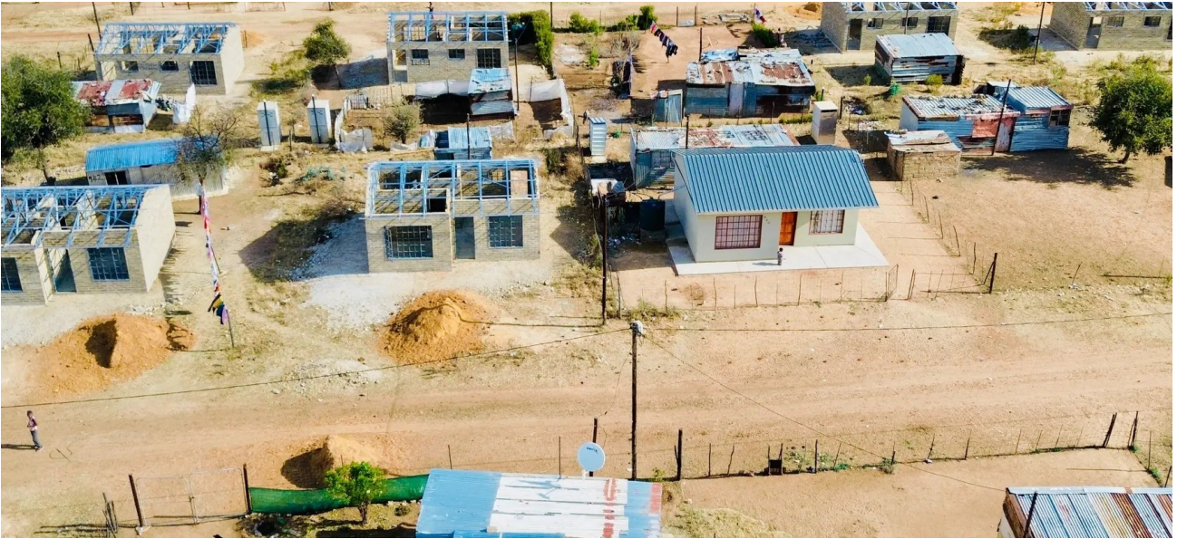
Aerial view showing simultaneous housing construction at different stages of completion
