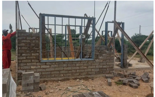
STRUCTURAL WALLING AND ROOF-FRAME PROGRESS
