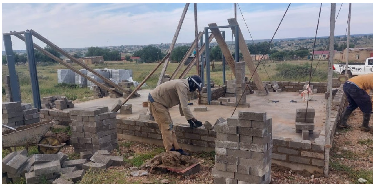
Housing construction in progress - building from foundation and structural stages
