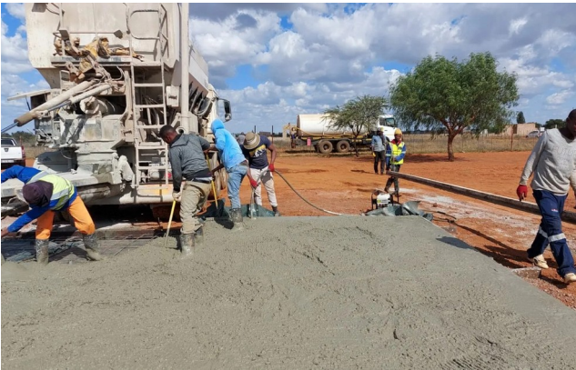
CONCRETE PLACEMENT AND FOUNDATION WORKS
