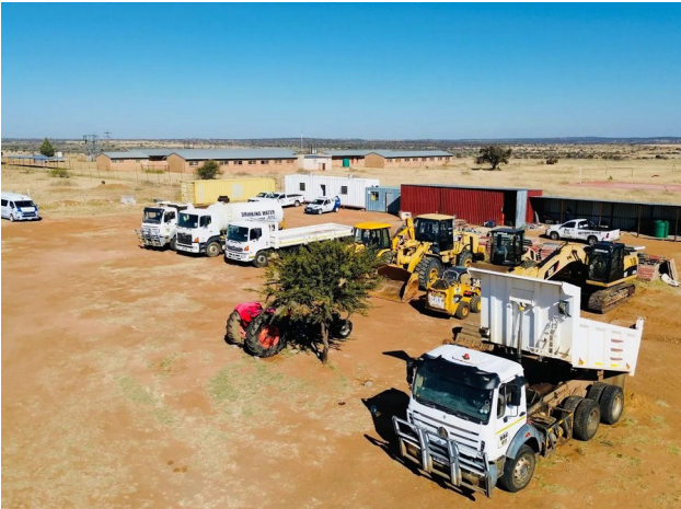
PLANT BASE AND EARTHMOVING FLEET
