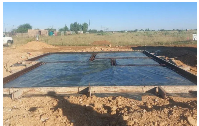
FOUNDATION AND CONCRETE WORKS
