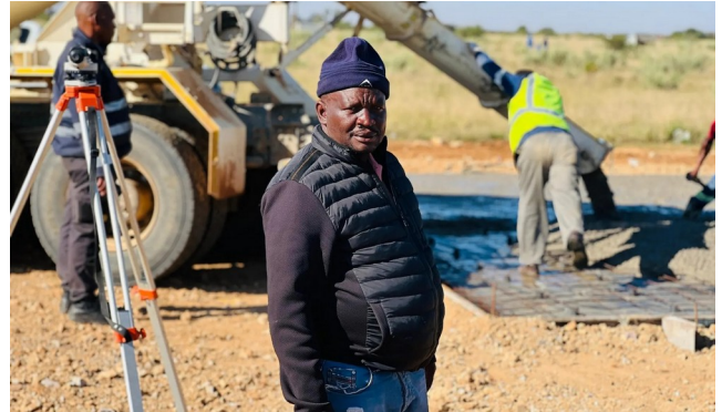
SURVEYING, SETTING-OUT AND QUALITY CONTROL ON SITE
