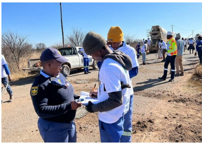
INDUCTION &amp; SITE COMPLIANCE
